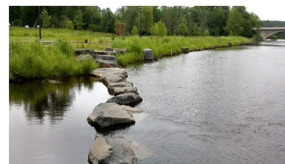
Natural shoreline restored, stone jetties create riffle habitat
